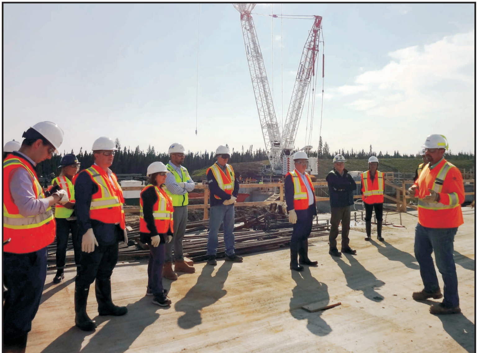
A tour group including multiple members of government and representatives from the AIOC checked out the Cascade Power Plant on August 26. Everyone was decked out in safety gear (see pages 16 and 17 for story and pictures). photo Shaylyn Thornton
