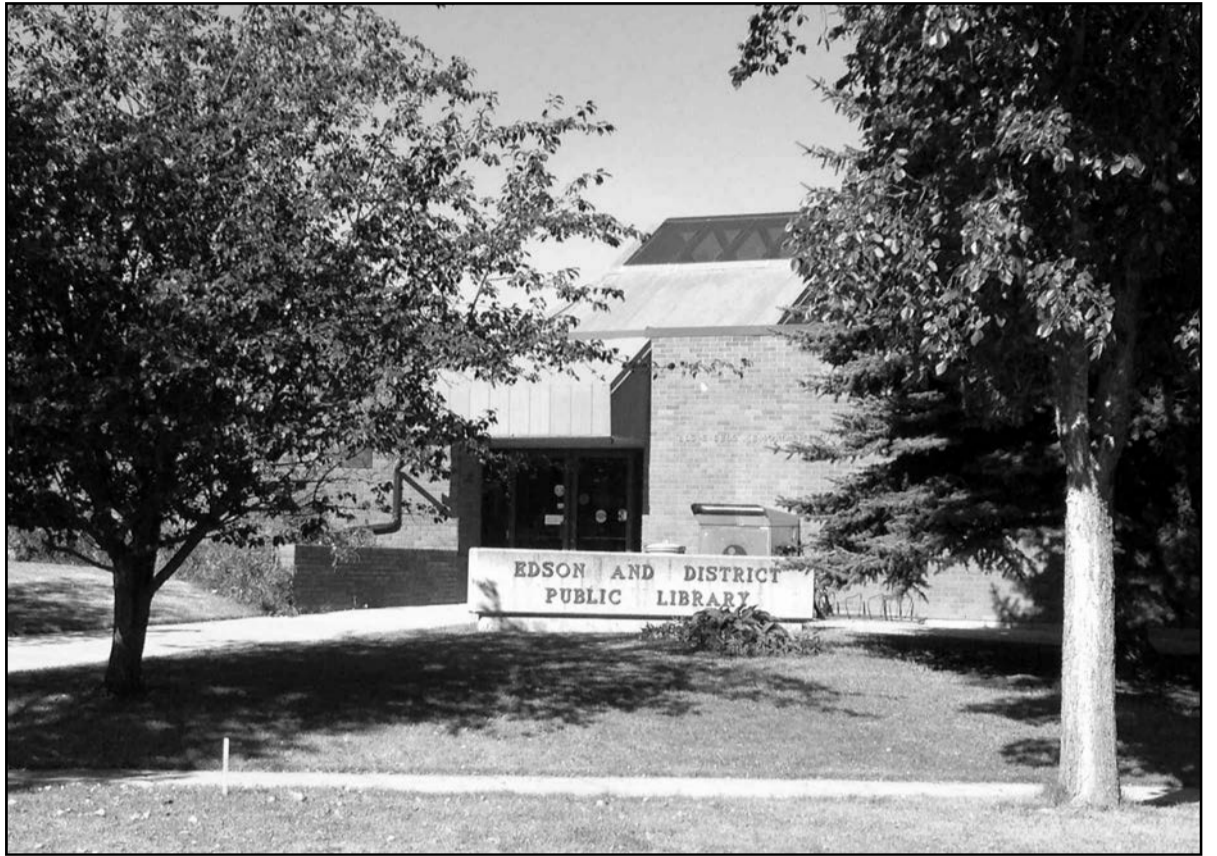
The Edson Public Library is look into a $2.2 million project that would see an expansion to the building.
