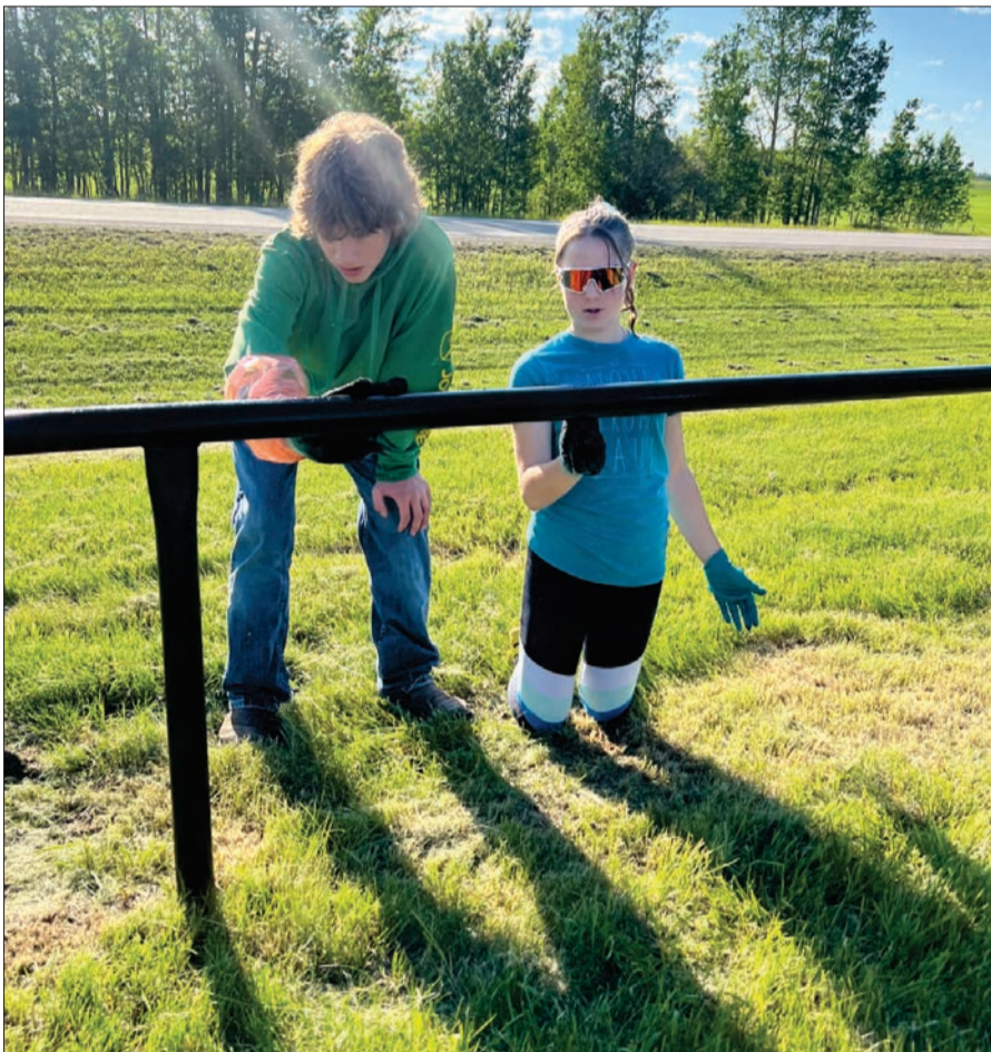
The Peers 4-H Multi Club volunteered to paint the new pipe fencing at the McLeod Valley Cemetery on June 19. submitted
