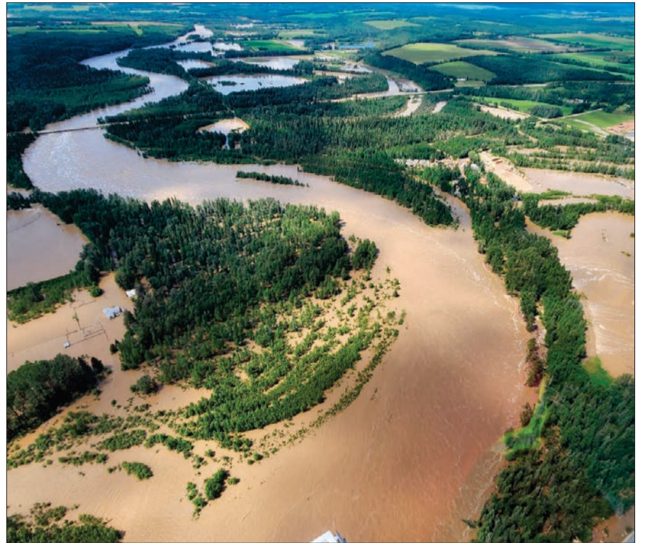
McLeod Valley in the foreground and Hwy 32 bridge in the background. Yellowhead County suffered extensive flooding due to heavy rains over several days as rivers and streams overflowed their banks. Many properties and homes were flooded leading to a local state of emergency on June 19.
